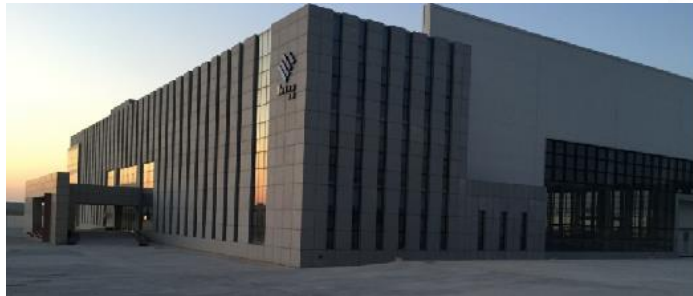
Shenyang Facility in China by LUSY
